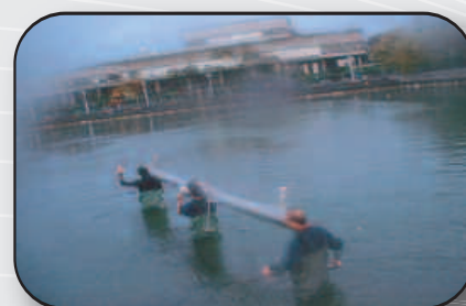
● Campion M&E engineers installing fountain.
