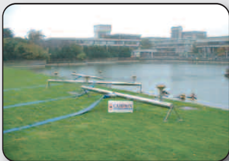
● Fountain ready to be installed.
